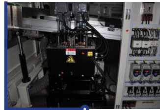
Solder pot inlet / outlet by motorized
